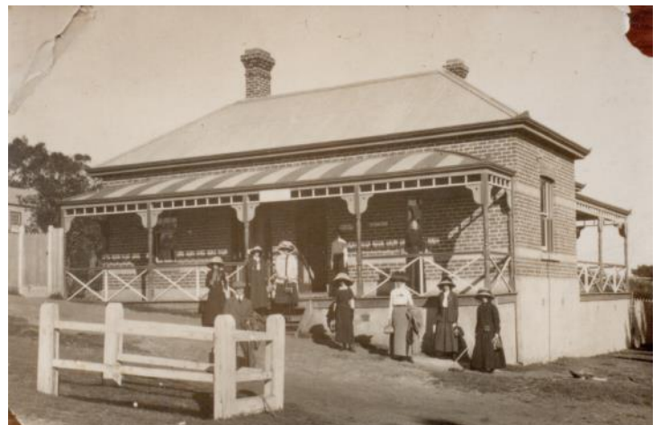
The building constructed from the bricks from the West's kiln which became the third Cowes Post Office.
